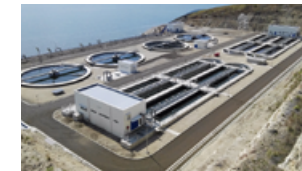
Sewage treatment plant
